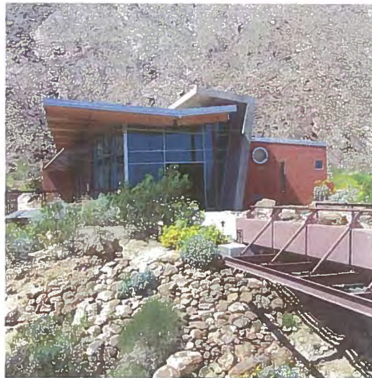
Tahquiltz Visitor Center : Entry Bridge
