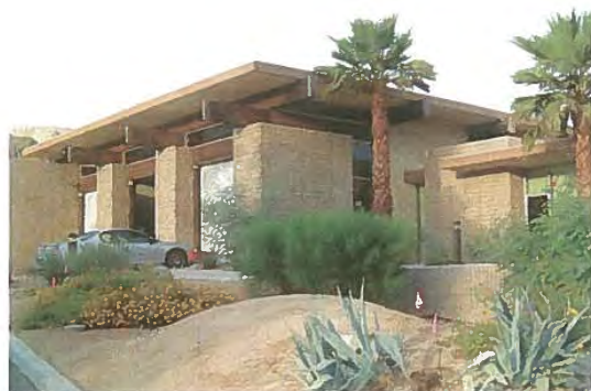
FIRE STATION 50 Renovation, Rancho Mirage, California
