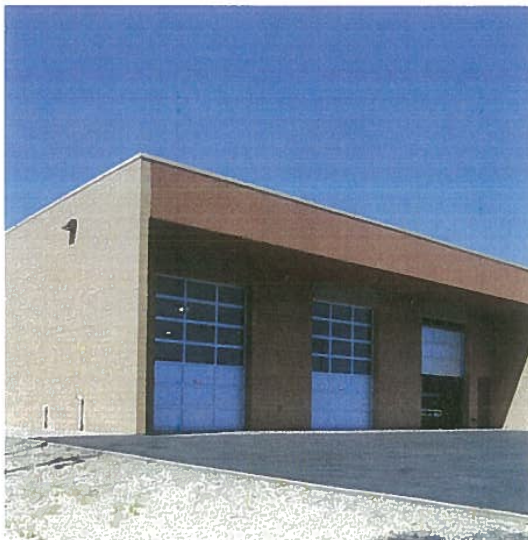
Desert Water Agency Maintenance Facility, Palm Springs, California
