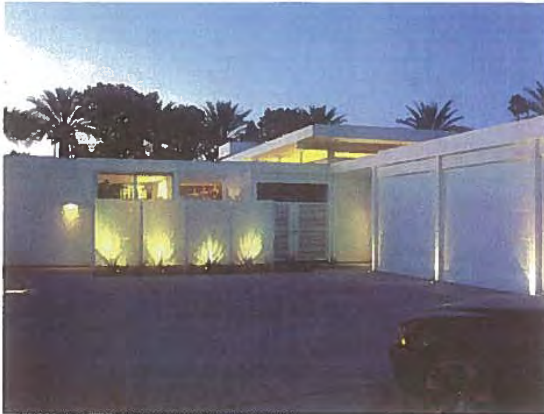
Zoll Residence. Motorcourt & Glass Screen
