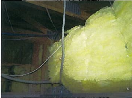
Photo 1.0 Existing Attic with R-30 Insulation (typical)
