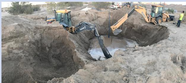
**Photo Caption:** All crews responded to a major water feed-line break at Well 14 that was located 30 feet deep! The repairs began at 9AM on August 6, and concluded at 4AM on August 7. Controlled shut-downs interrupted water service to a few customers, and impacted water pressure to many others.
